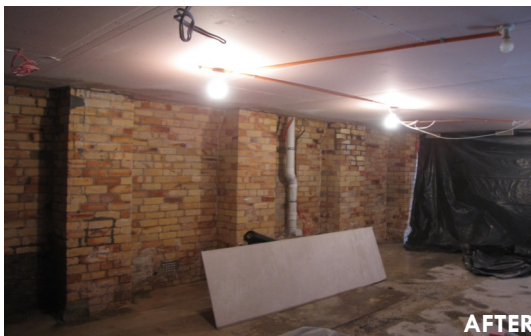
Now ready for waterproofing
