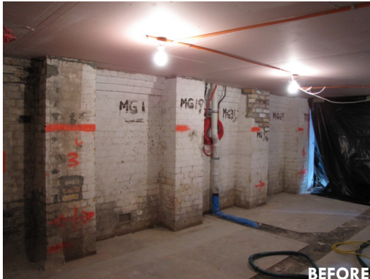
Commercial basement—Howe St.—Auckland
