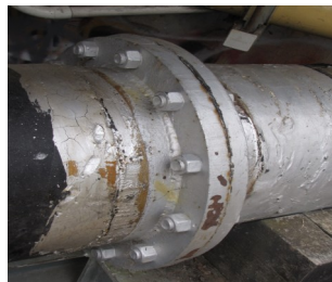
Water main junction cleaned up for inspection & recoating
