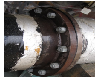
Water main junction cleaned up for inspection & recoating
